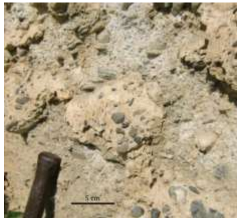
Fig. 9 CH2. Superficial oxidation and desquamation.
